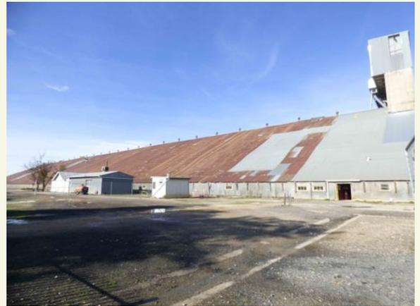
This structure was built in 4½ months, ENTIRELY by manual labour. Work commenced on 25<sup>th</sup> September 1941 and the store was ready to receive wheat in January 1942. The first wheat in BAGS was delivered on 22 January 1942. The first railway truck of bulk wheat arrived on 17<sup>th</sup> February. It was the beginning of bulk storage. The capacity of storage was 95,000 tons.
