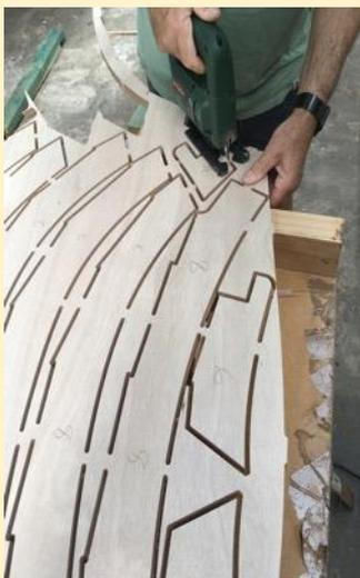
*The kit consists of CNC cut plywood and some additional wood to shape and fit*
